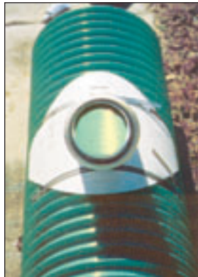
11. Properly align saddle with saddle gasket to prevent obstruction of incoming flow.
