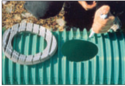
7. Apply silicone to the O.D. of Ultra-Rib around the tap hole as shown.
