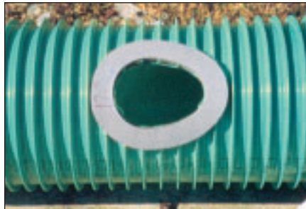
9. Place saddle gasket over the tap hole as shown.
