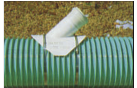
12. Attach two stainless steel bands as shown.
