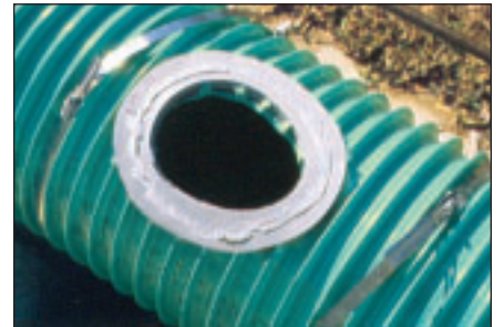
10. Apply silicone in a continuous bead (as shown) to the smooth side of the gasket.
